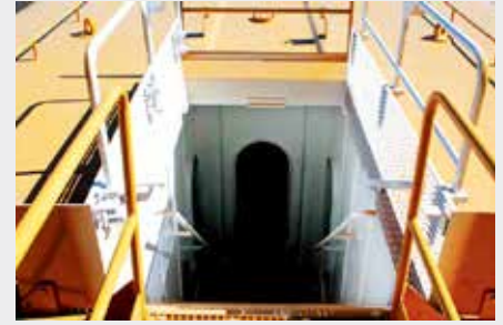
Stairway access down inside the water tank
