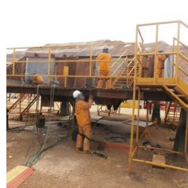
On-site maintenance and shutdown services (Pilbara Hire)
