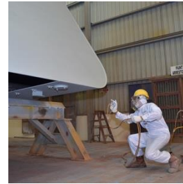
Painting and blasting
