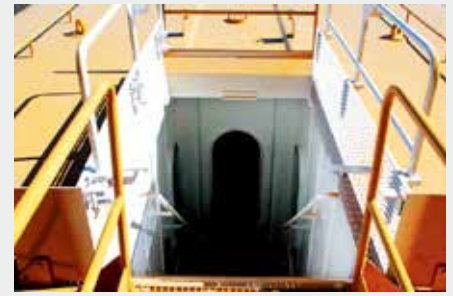
Stairway access down inside the water tank
